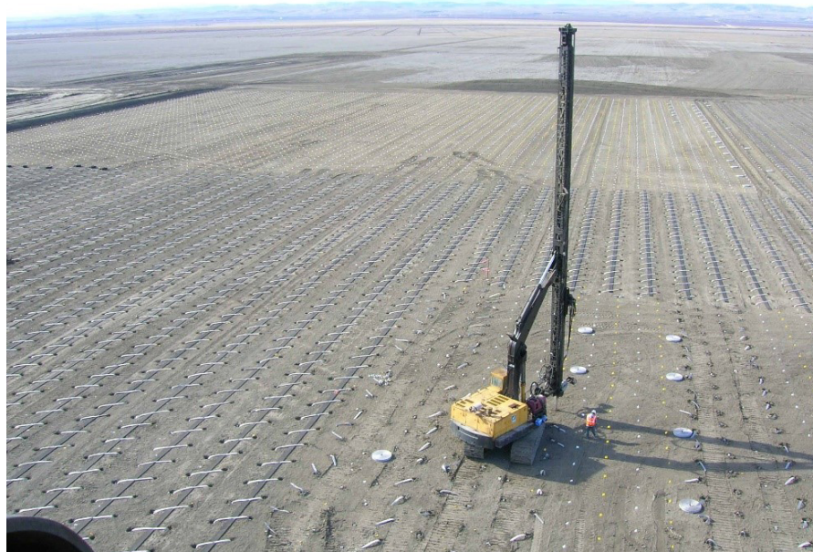
Courtesy Menard Group USA Figure 2-6. Strip drains.
