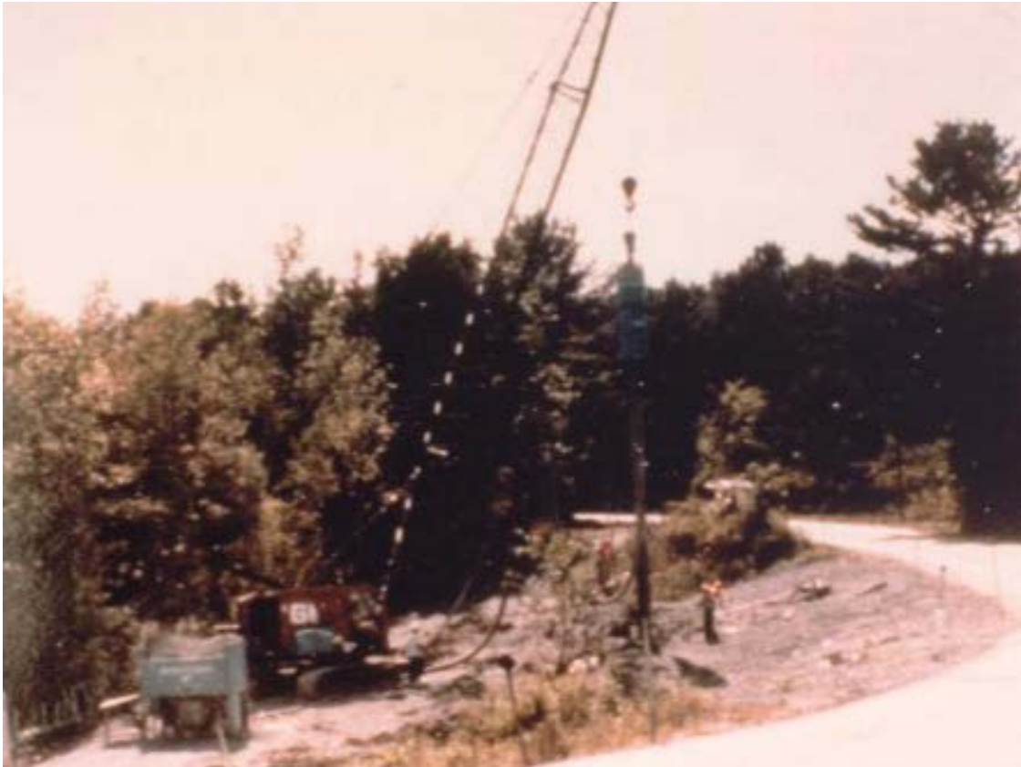
Figure 5-30. Stone column installation.
