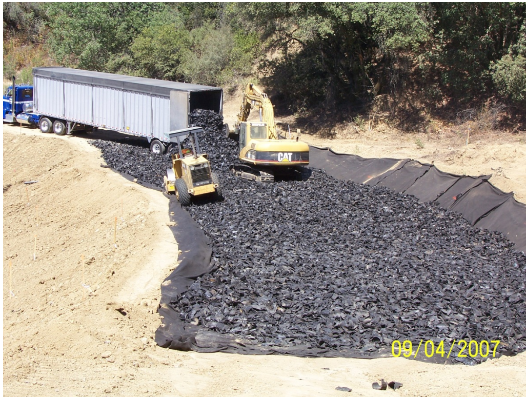
Figure 3-16. Placement and compaction of TDA within geotextile wrap.
