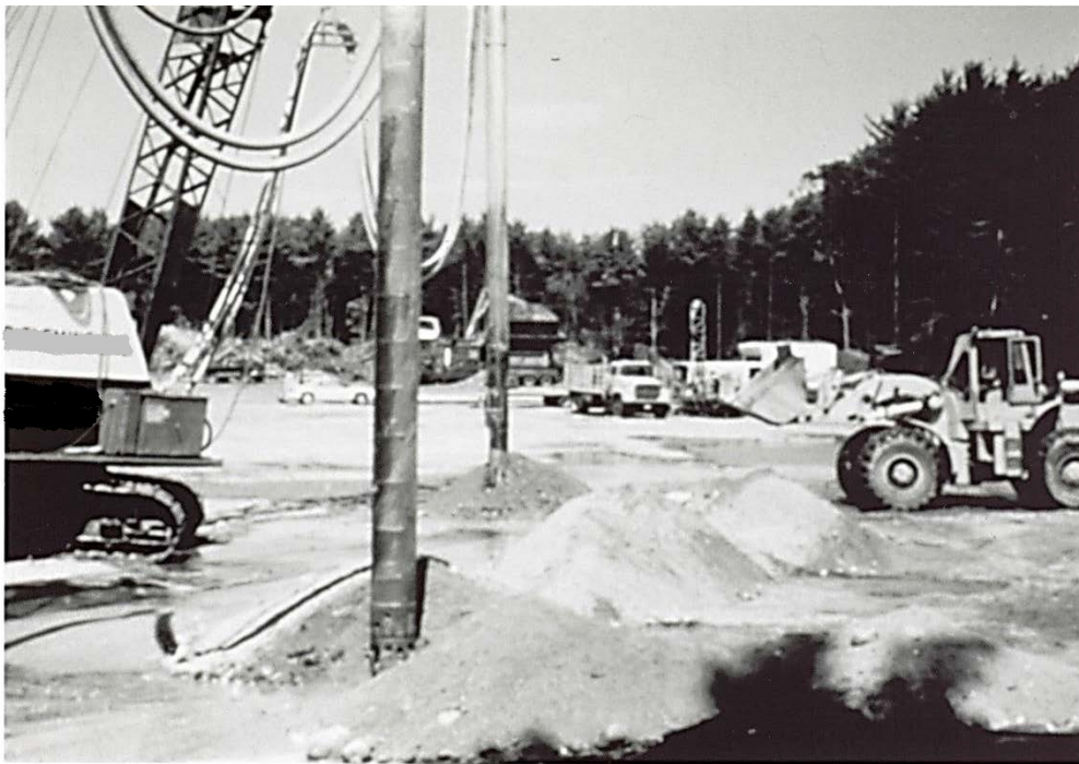
Figure 4-31. Vibrator suspended from a conventional crane.
