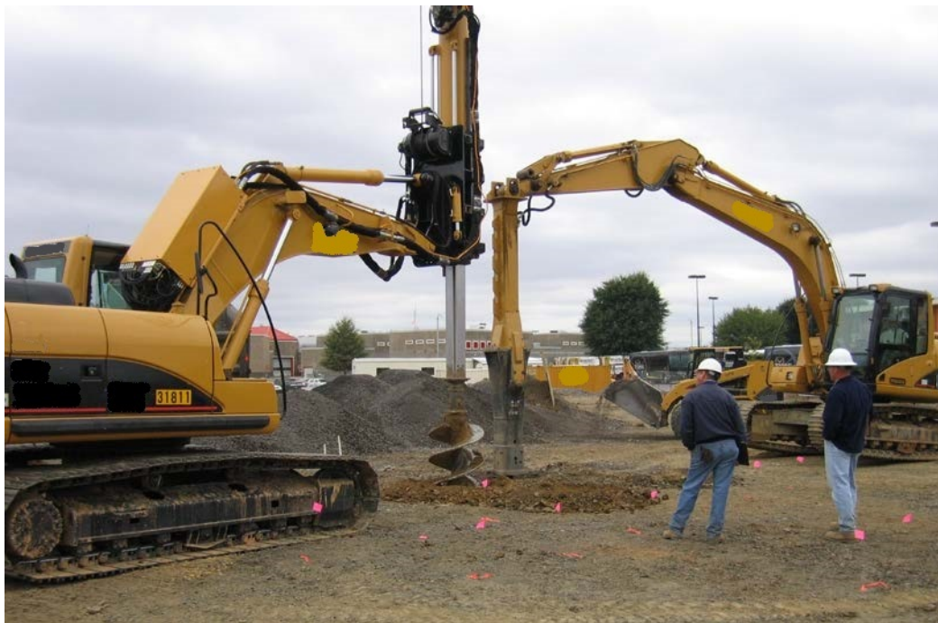
Figure 5-15. Replacement method, rammed aggregate pier with predrilling.
