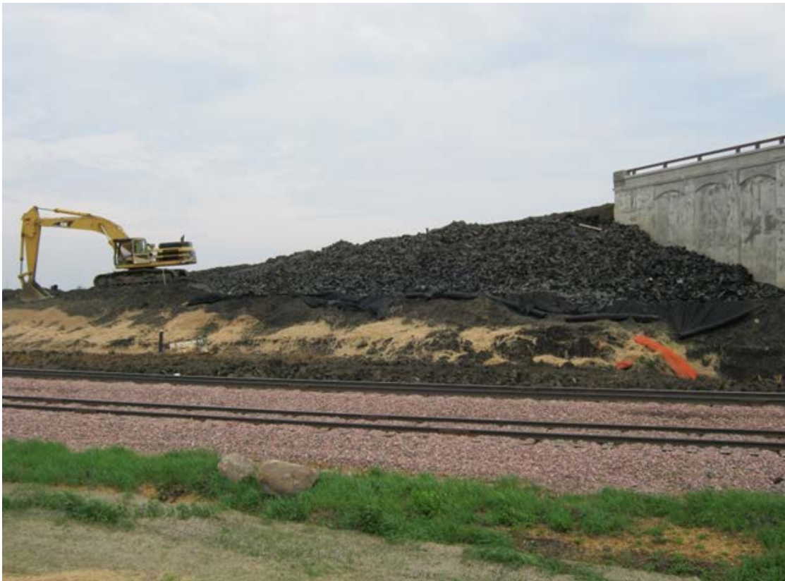
Figure 3-3. Embankment fill construction with tire shreds in Blue Earth County, Minnesota.
