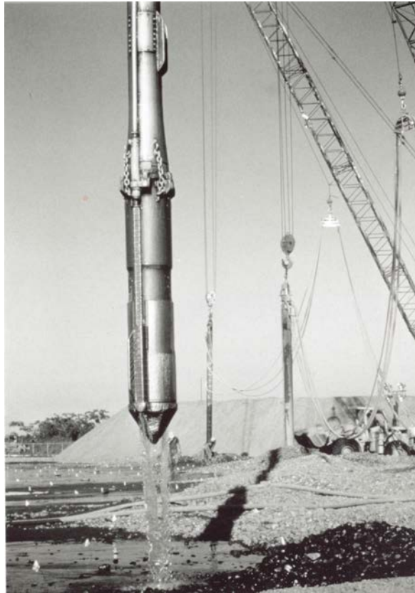
Figure 5-4. Suspended vibrator.
