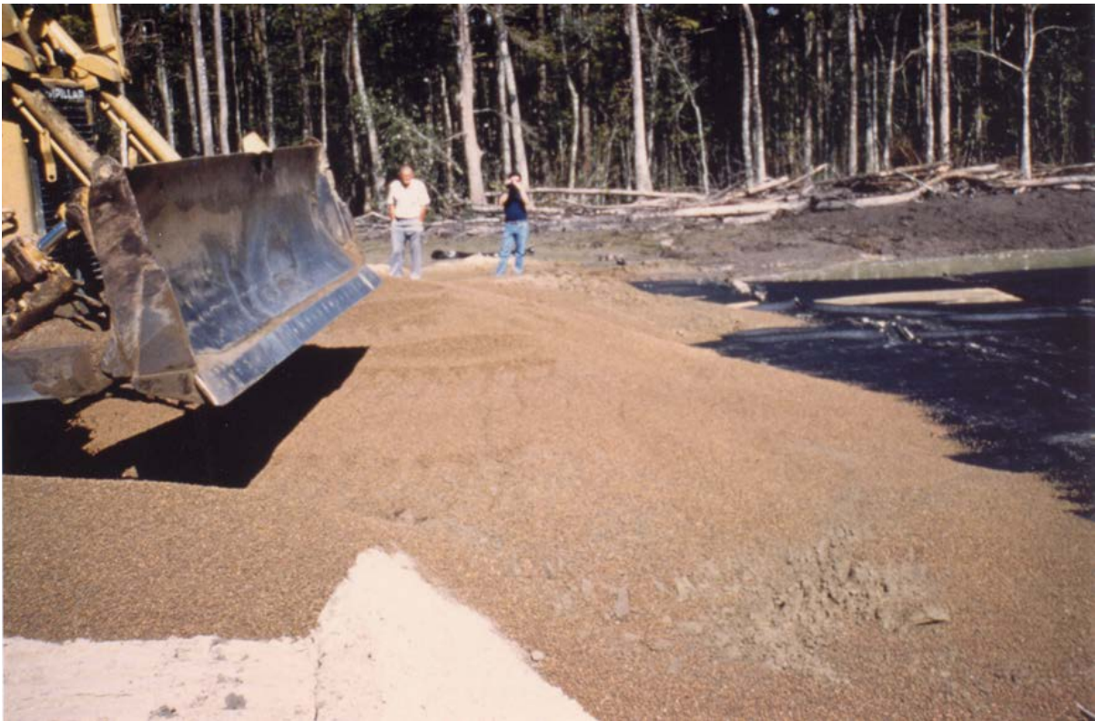
Figure 3-5. Placing expanded clay fill.
