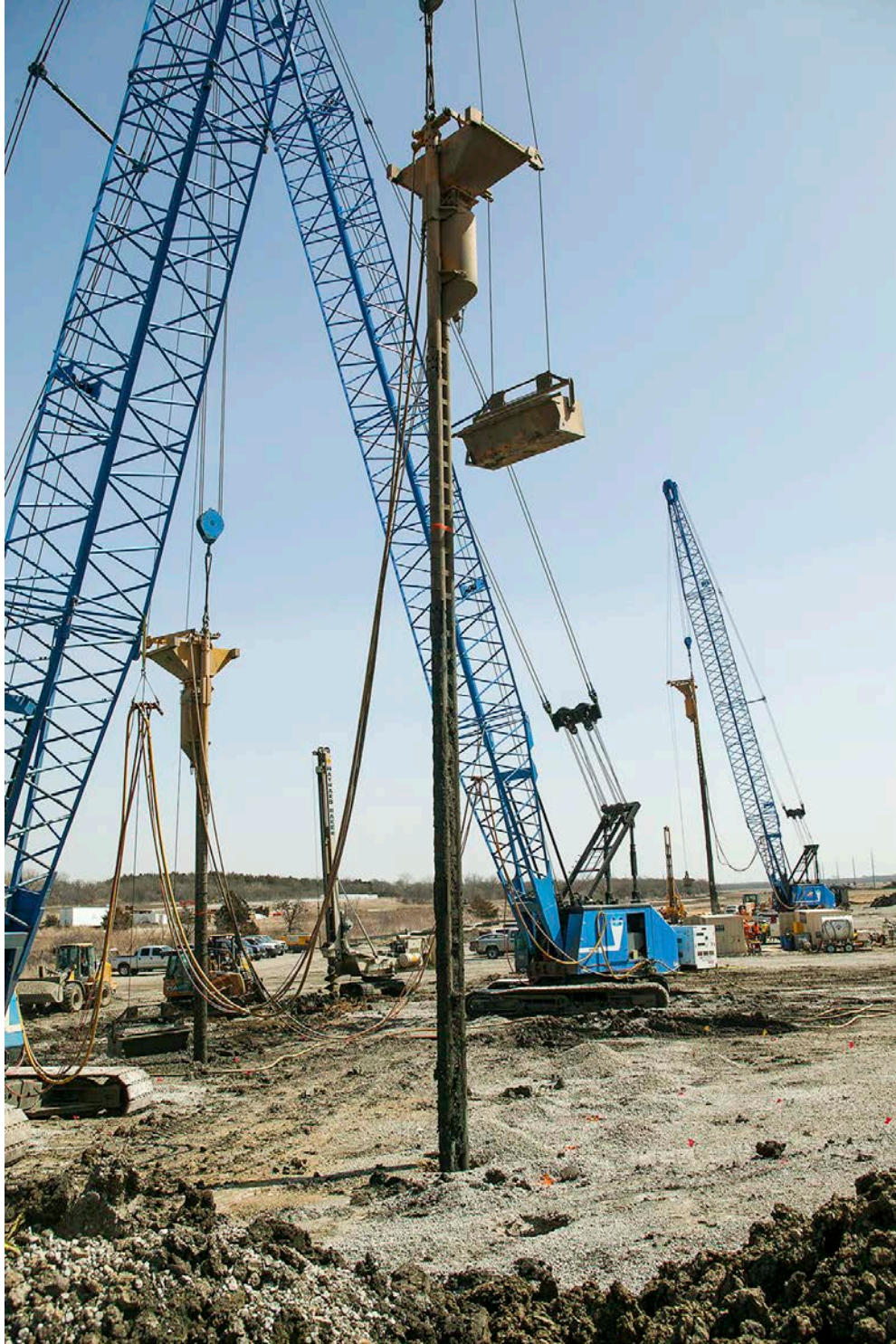
Figure 5-7. Stone column dry bottom feed rig.
