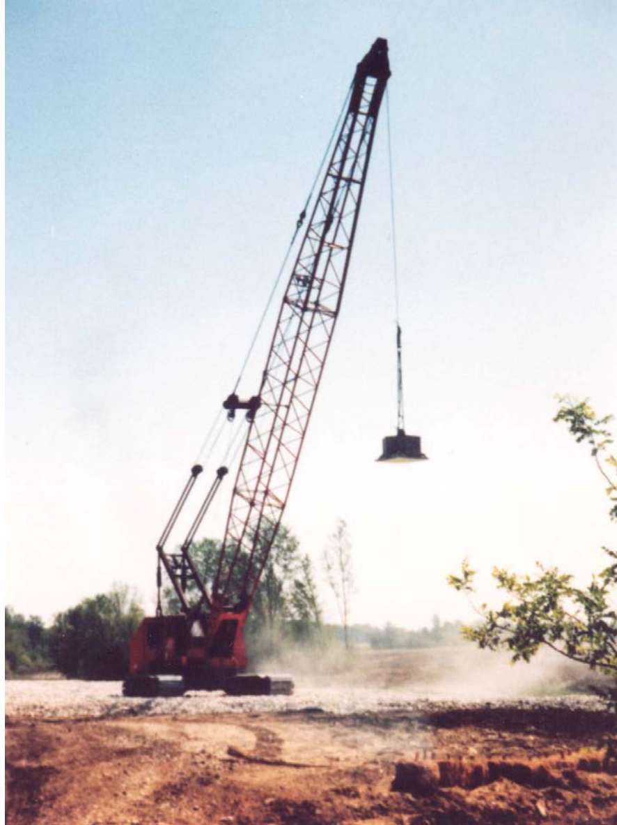
Figure 4-20. Deep dynamic compaction over a 3-foot layer of crushed rock placed on a landfill.
