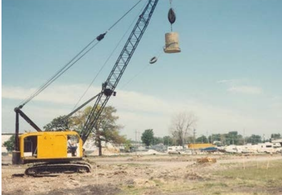
Figure 4-15. Lifting crane of 70 kips rated capacity used with 12 kip tamper.
