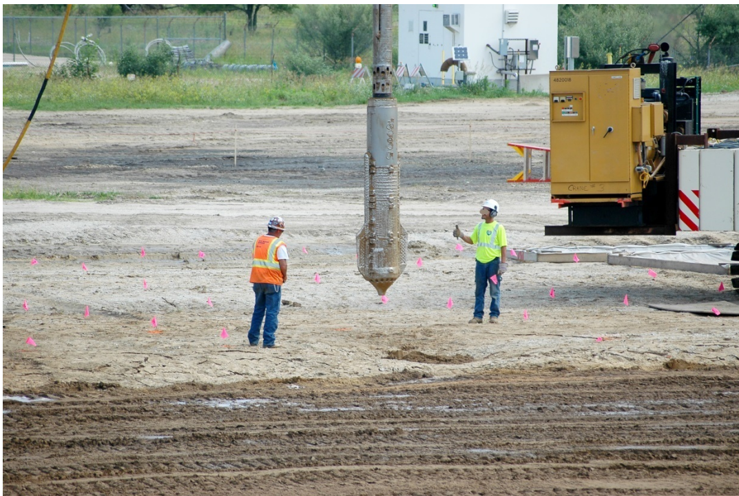
Figure 4-29. High-powered, probe-type vibrator utilized in vibro-compaction.
