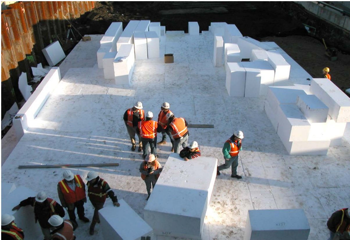
Figure 3-1. Embankment construction with EPS-block geofoam.
