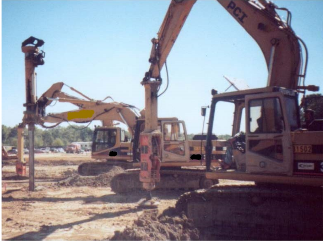
Figure 5-14. Rammed aggregate pier tamper.
