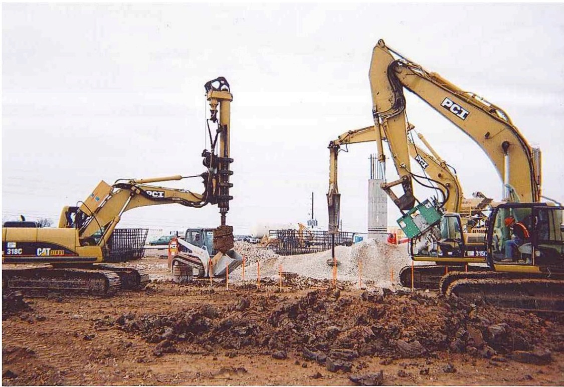
Figure 5-28. Rammed aggregate pier installation.
