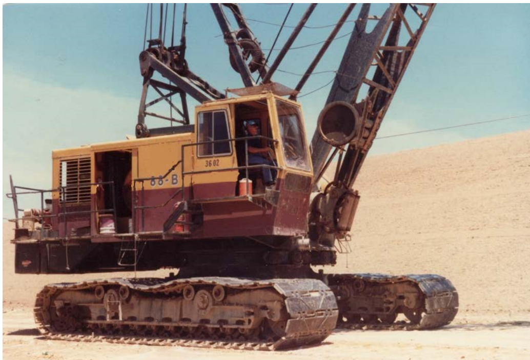
Figure 4-16. Dragline-type lifting crane with 1¼-inch cable for use with 40 kip tamper.
