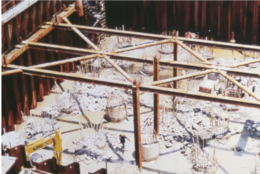
Figure 10 - Cofferdam for the Sidney Lanier Bridge, Oregon
