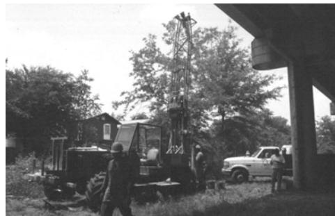
All-Terrain Rotary Drill Rig with Donut Hammer
