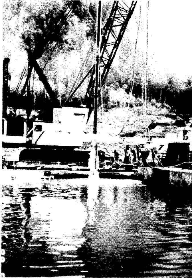
Figure 6. Vibrator suspended from a barge-mounted crane.
