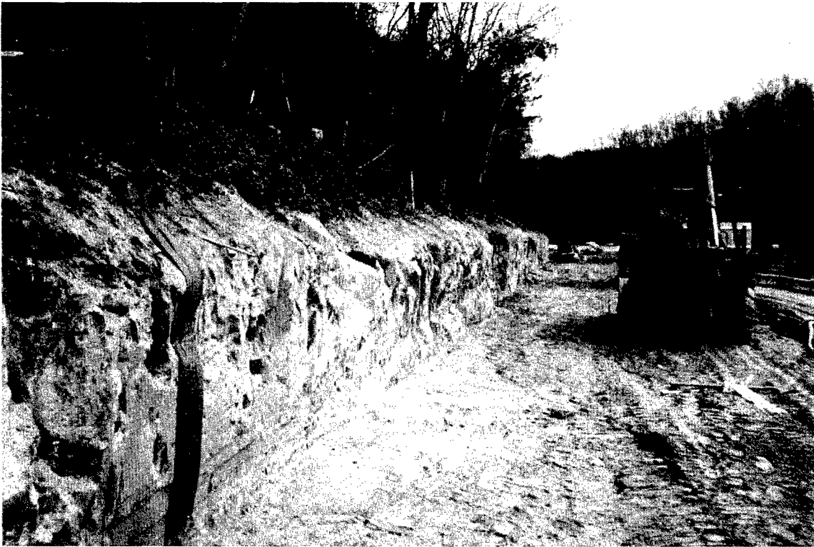
Figure 2. Excavation of first lift and placement of drainage strips.
