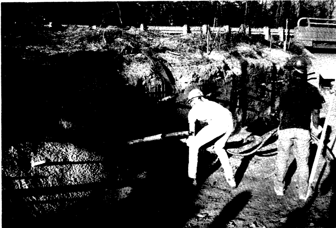
Figure 5. Grouting a nail hole.
