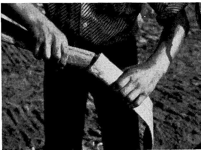
b. Inserting the drain core within the jacket to maintain continuity
