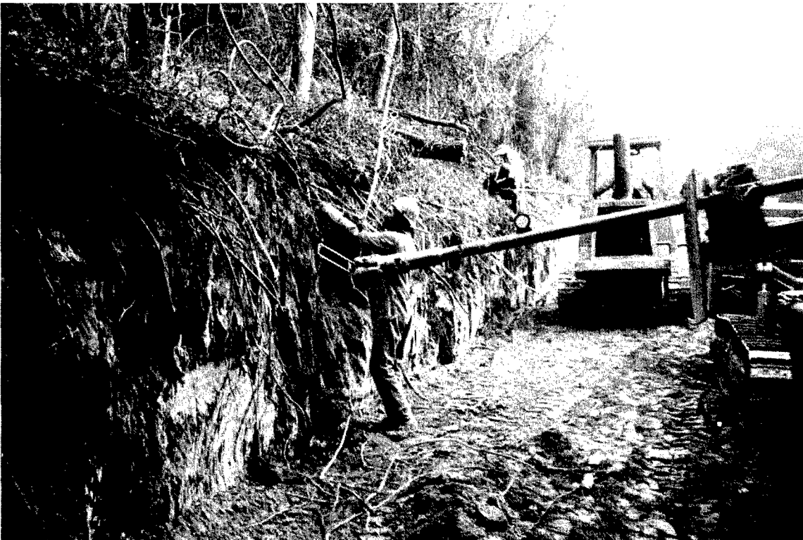
Figure 3. Drilling a nail hole.
