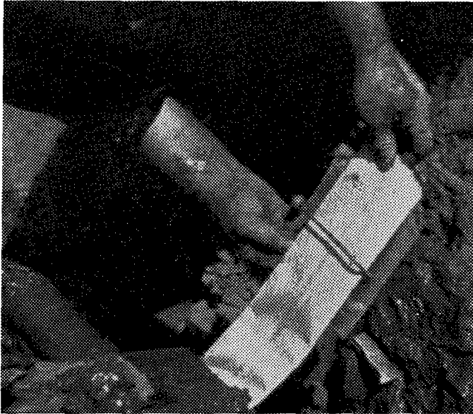
a. Placing the anchor on the drain
